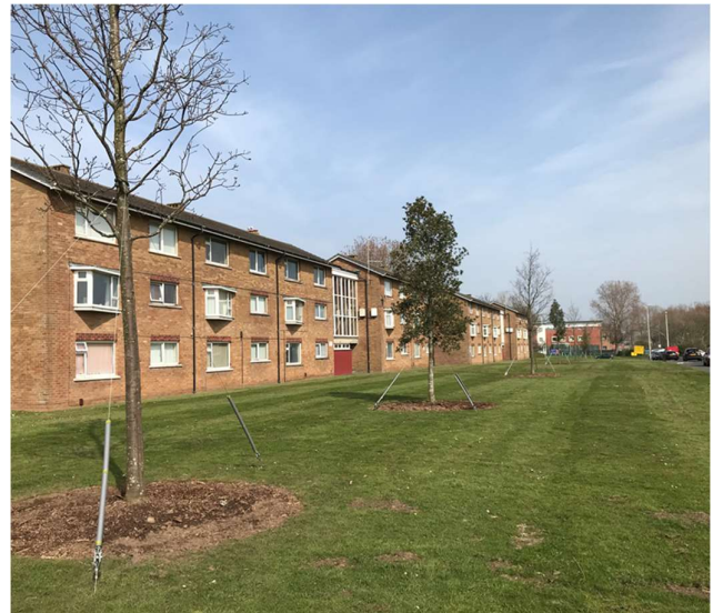
Figure 4. Tree guying on Munster Avenue, Bispham
